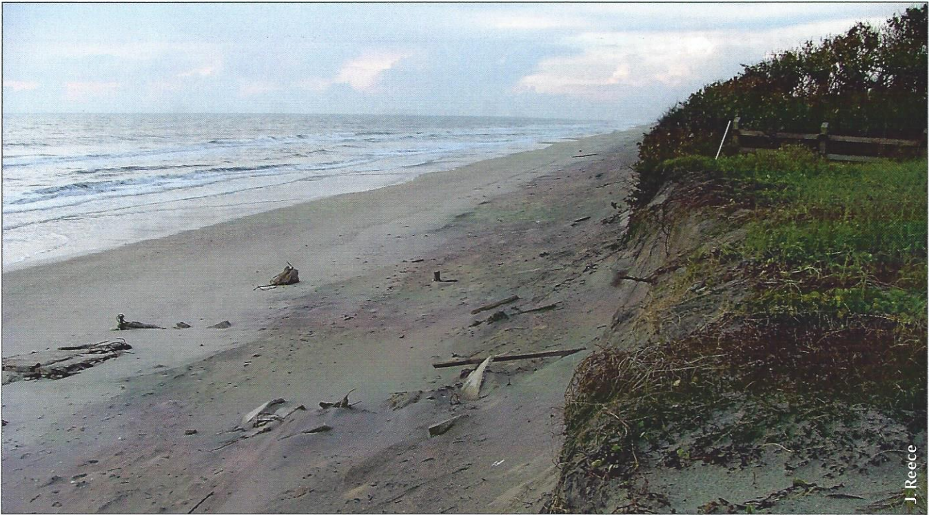
Eroded parts of the refuge (Melbourne Beach, Florida)
